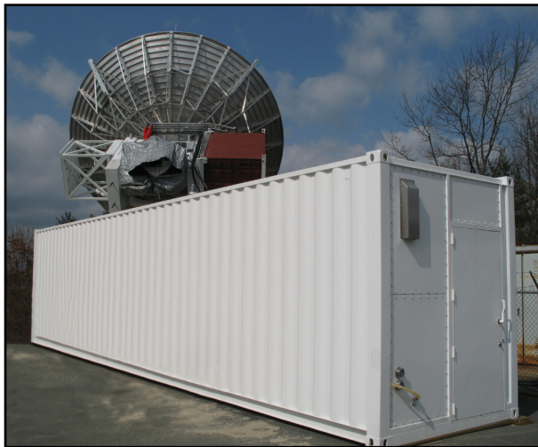
Transportable Shelter housing X-band Transmitter Components. This weatherproof shelter contains a high-power RF amplifier, two 200 kW high voltage switching supplies, capacitor bank, power distribution unit, transmitter controls, environmental controls, and cooling/air conditioning systems.
