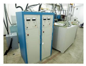
Figure 2. Installation of the 2 MW klystron transmitter. View shows DTI's high voltage power supplies (left) and capacitor tank (right).
