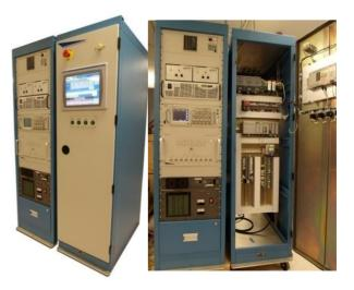
Figure 5. Controls racks for the 2 MW klystron transmitter.
