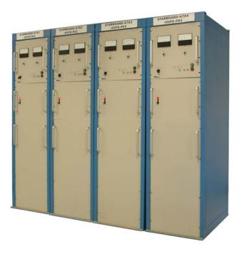
Figure 7. Four, 45 kV 150 kW switching power supplies drive one of two 8-TWT groups. The power supplies in each group have N+1 redundancy, allowing full power operation if one supply is off-line.
