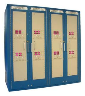
Figure 6 Eight TWT modulator assemblies are located in these cabinets. The eight TWT cathodes will be located directly above this cabinet in the final installation. Each modulator assembly has its own fault control panel as shown in Figure 9.
