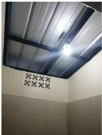
Here are pictures of the new roof at Villa Lora. It has steel beams and 40 year aluminum roofing.
