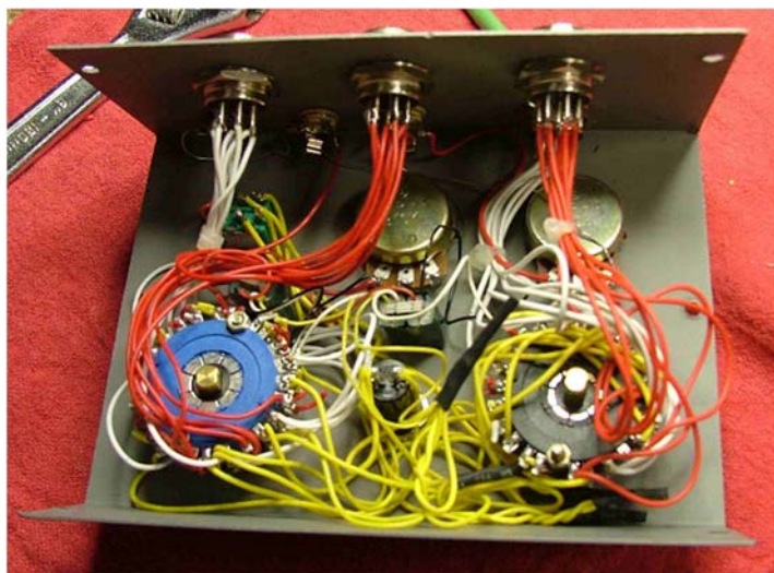
Inside wiring and part placement
