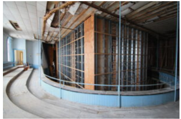
The balcony of the Norway Opera House. The roof is supported by a series of supports put in place in 2011.
