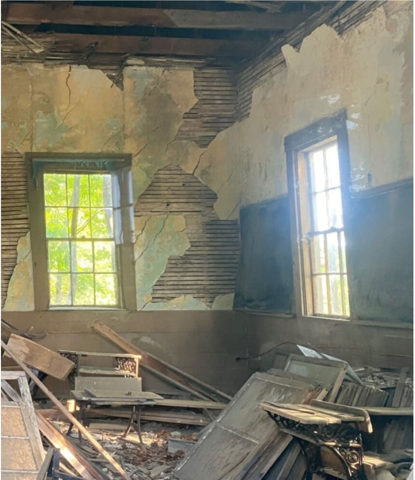
The 1987 Pigeon Hill Schoolhouse on Route 26 in Oxford has no ceiling, broken plaster walls, broken desks, a stack of old windows and other debris. The Oxford Historical is trying to save the town's last standing one-room schoolhouse by moving it to its headquarters in the village and restoring it as a living history museum. Nicole Carter/Advertiser Democrat
