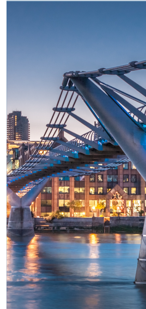
Tour Millennium Bridge
