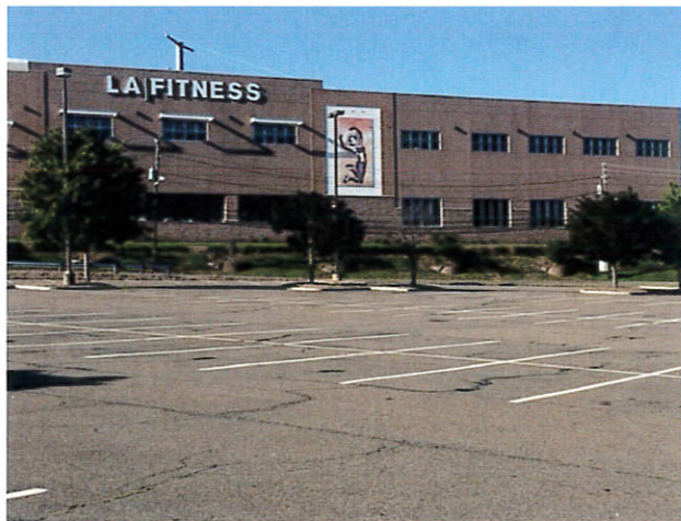
LA Fitness located south of the site.
