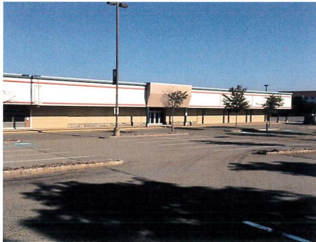
Façade view of Building B.
