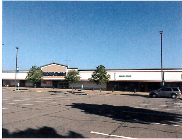
Façade view of Building A.
