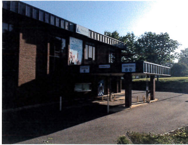
Building F: Existing bank with drive-through lanes.
