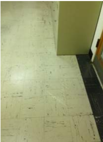
A21 _Test flooring tiles and replace/cover at lower level storage/stack area
