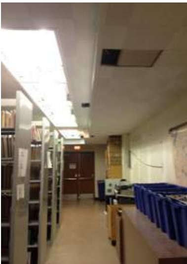
A23_Replace ceiling at lower level storage/stack area
