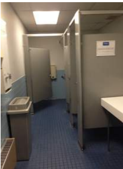
A29 _Modify public restrooms for ADA compliance
