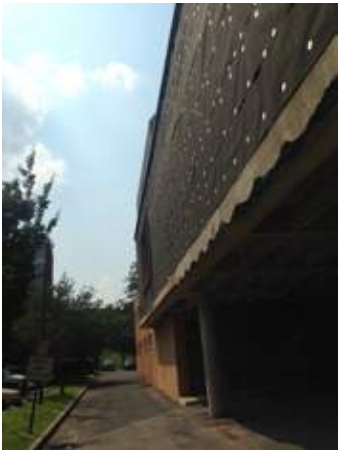
A1 _Brick facade replacement at 1978 addition
