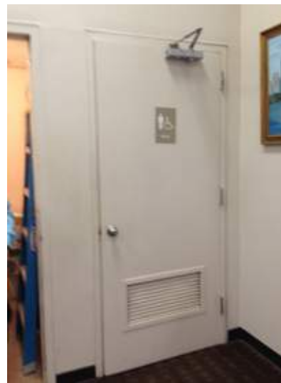
A28_Modify public restrooms for ADA compliance
