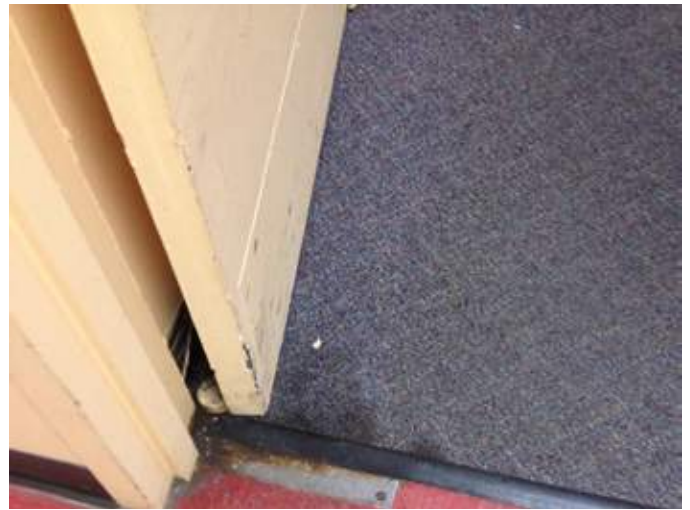
A26 _Paint walls and replace wall base at lower level storage/stack area
