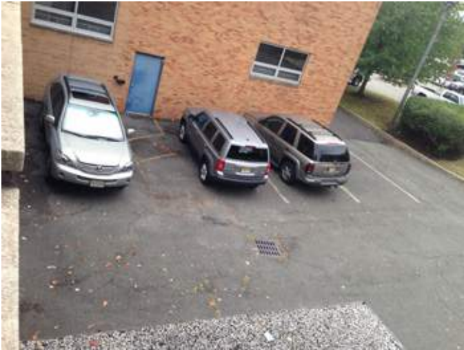
A16 _Side driveway and staff parking lot - seal coat and restripe
