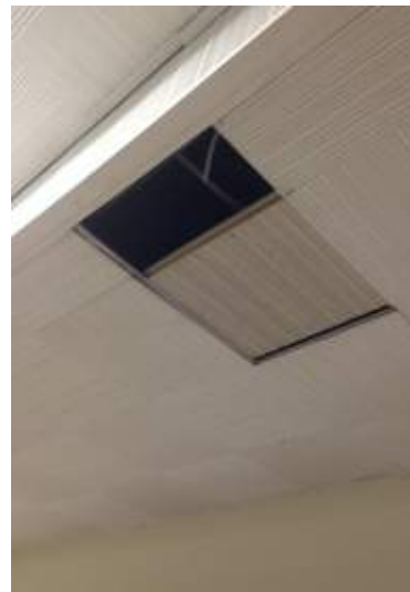
A24_Replace ceiling at lower level storage/stack area
