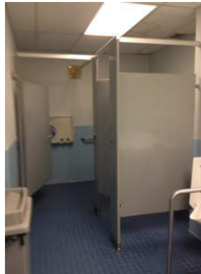
A30 _Modify public restrooms for ADA compliance
