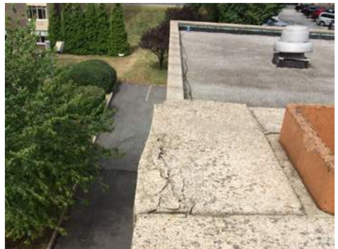
A6 _Chimney cap stone replacement and flashing
