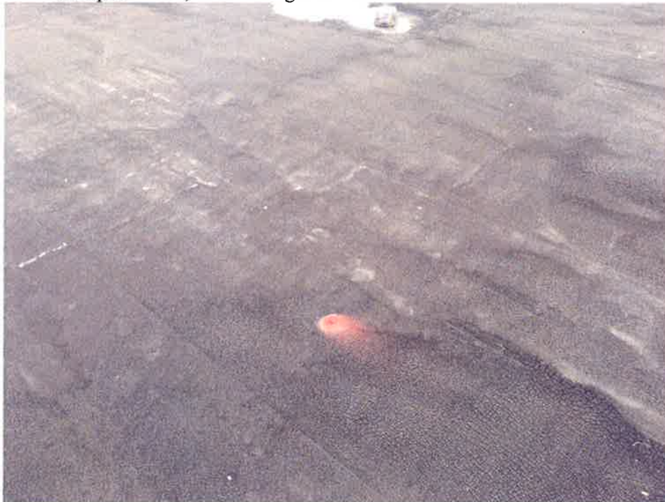
#2 – Detail of Sample site 09; Black shingle/tar- confirmed as ACM
