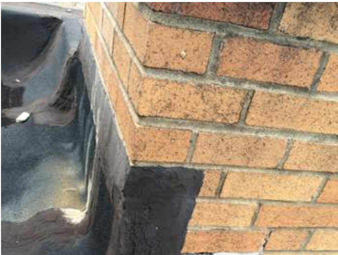
A7 _Chimney cap stone replacement and flashing
