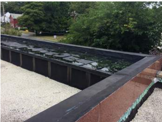
A5 _Roof replacement and new coping at original building
