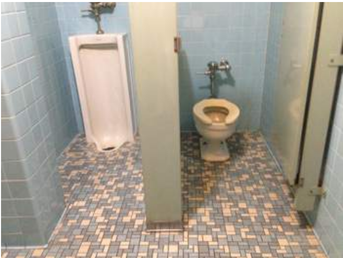
A31_ New plumbing fixtures and accessories at all other restrooms
