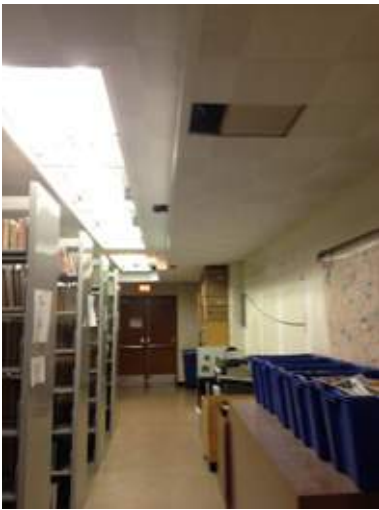
A25 _Paint walls and replace wall base at lower level storage/stack area
