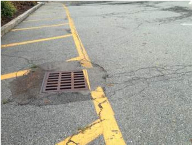
A15 _Gaston Street parking lot - mill and repave, restripe, proper ADA signs and layout
