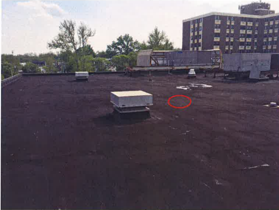
#1 – Overview of 1979 addition roof; Site of sample 09 circled
