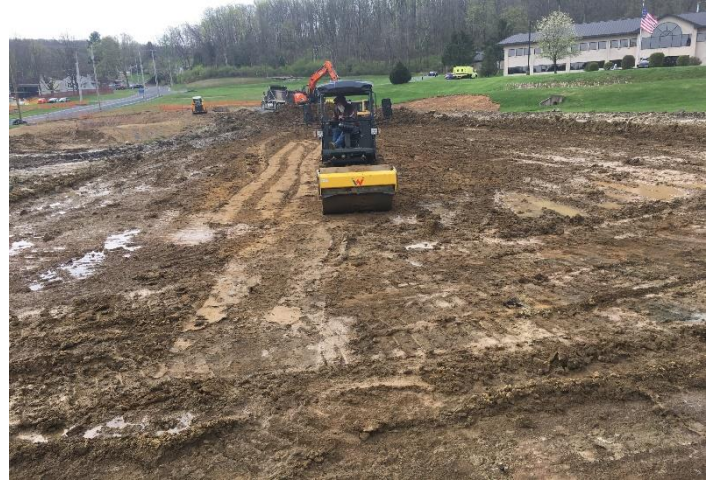
FIRE STATION PAD / GRADING & COMPACTION
