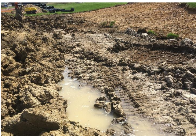
TOP FROM LEFT TO RIGHT: 1 & 2 IDENTIFIED AS A STREAM CROSSINGS TO BRING WATER ON PAD 3, 4, 5 & 6 IDENTIFIED AS WATER TRAPPING BEHIND STOCKPILING EXCAVATED MATERIALS
