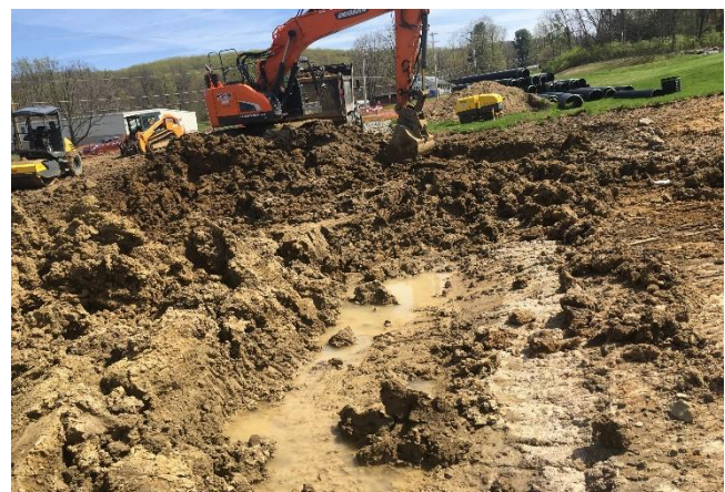
TOP FROM LEFT TO RIGHT: 1 & 2 IDENTIFIED AS A STREAM CROSSINGS TO BRING WATER ON PAD 3, 4, 5 & 6 IDENTIFIED AS WATER TRAPPING BEHIND STOCKPILING EXCAVATED MATERIALS
