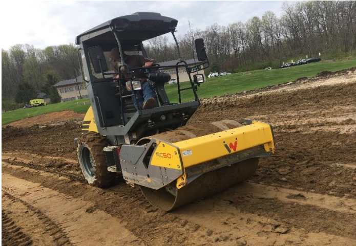
FIRE STATION PAD / GRADING & COMPACTION
