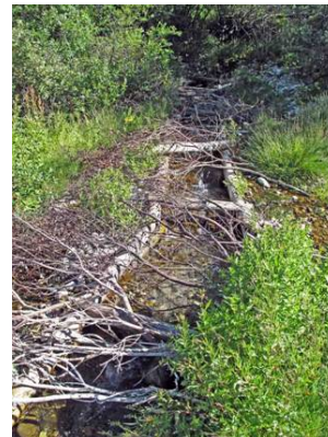
Above: This is a 2011 photo of the new spawning channel, ten months after its construction. Willow plants were placed along the edge of the log retainer walls and they will eventually hide most of the channel!
