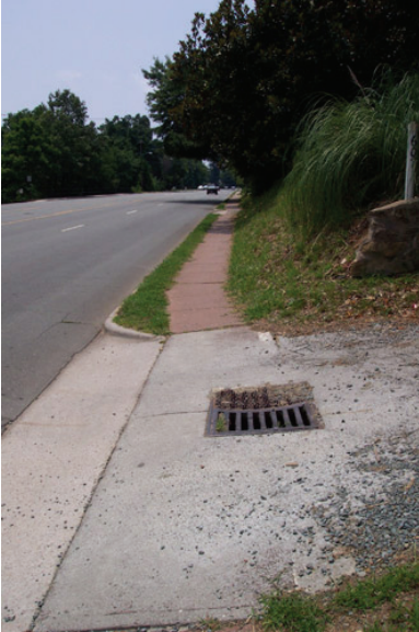
A drainage grate becomes a hazard for bike tires. Photo courtesy of www.pedbikeimages.org / Reed Huegerich.
