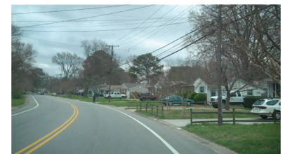
The new edge stripes along Aragona Boulevard left a paved shoulder suitable for cycling and walking.
