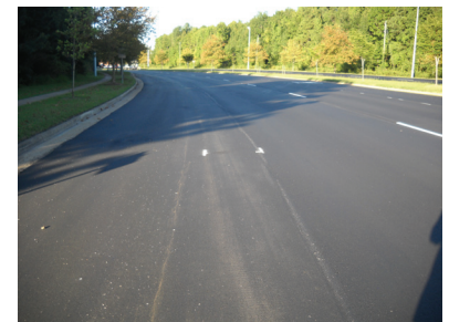
Dam Neck Road in the process of being restriped with bike lanes.
