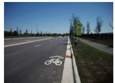
Signed Shared Roadway (with share arrow symbol). Photo courtesy of www.pedbikeimages.org / Heather Bowden
