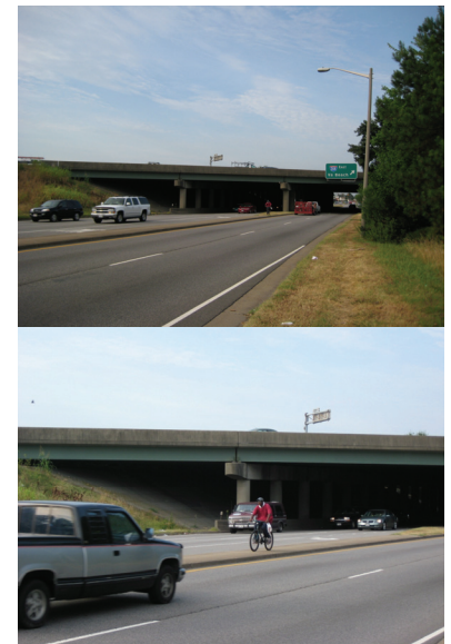
A cyclist struggles to navigate the underpass at Newtown Road.
