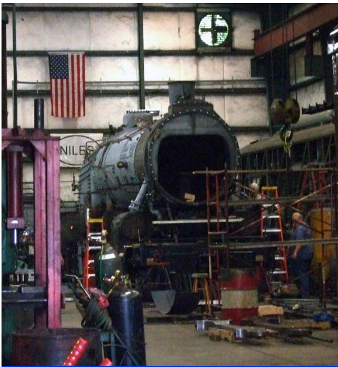
Restoring Another One
