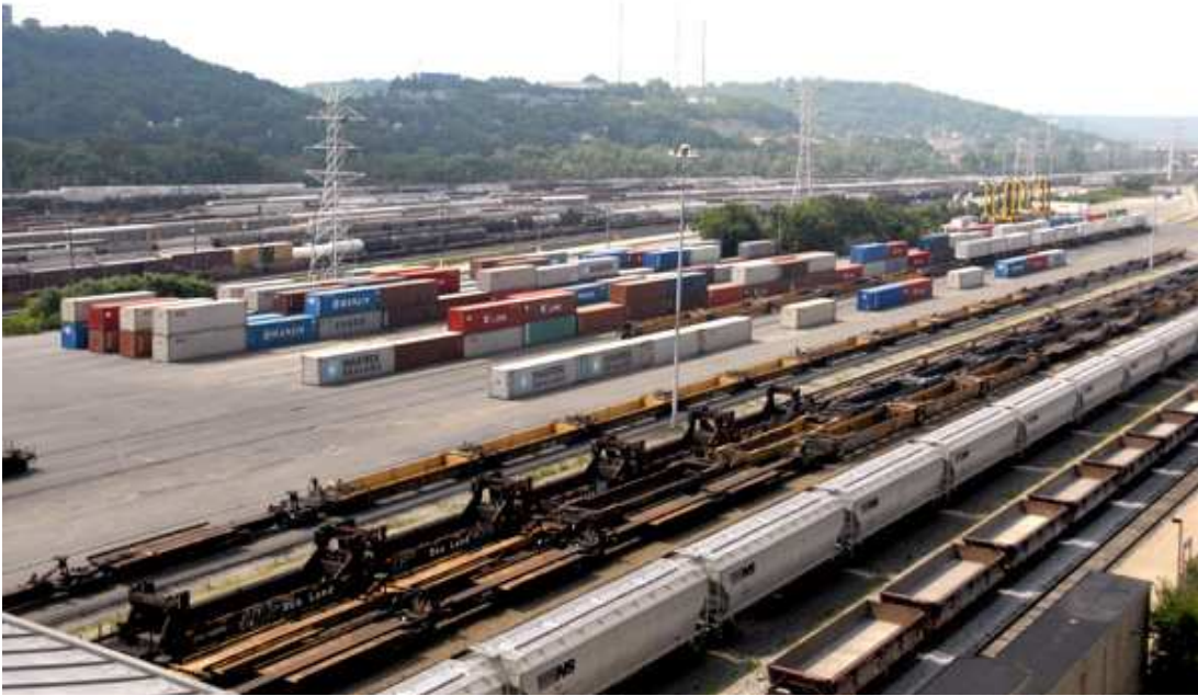
The Container Yard
