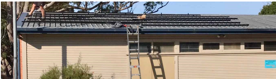
Solar panel installation in progress
