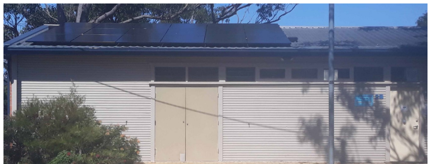
Installation of solar panels complete
