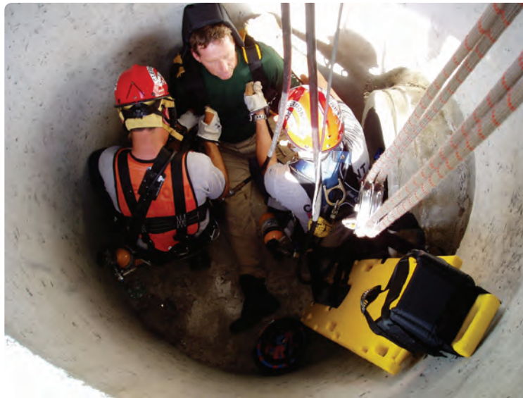
Fig. 32-7: Confined spaces include any space with limited access that is not intended for continuous human occupancy. Photo: courtesy of Chief Carle L. Bishop, Clermont Fire Department.
