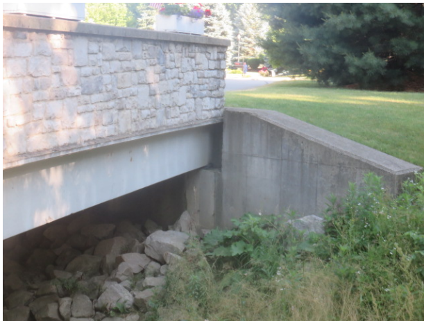
Concrete bridge abutment in good condition
