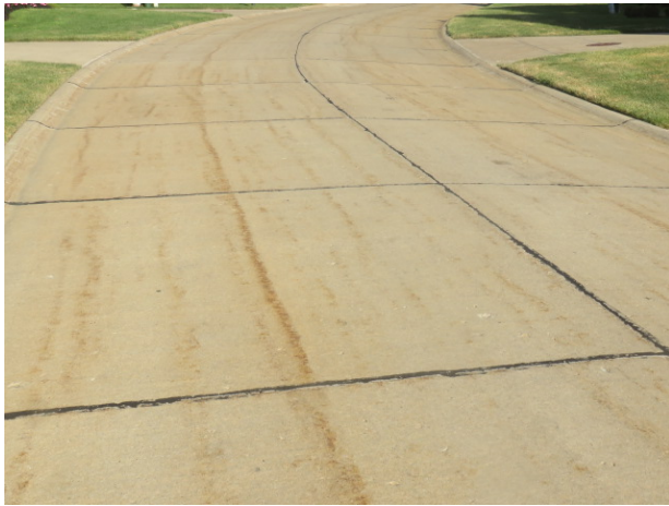
Concrete street overview
