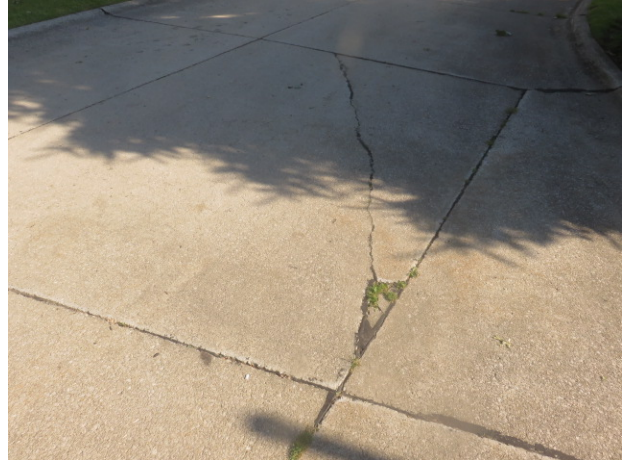
Unrepaired crack
