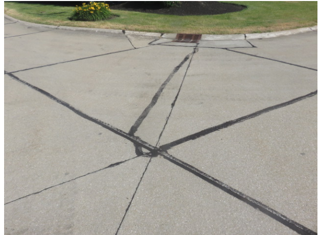
Repaired cracks at intersection near catch basin
