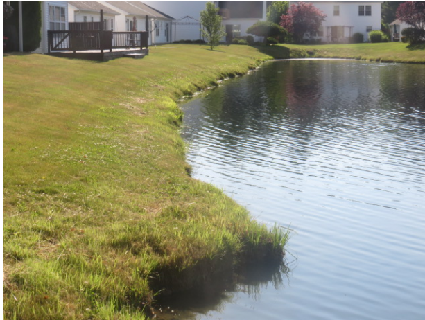
Shoreline and sloped embankment at north bank of pond
