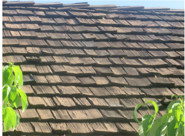
Cedar shake roof in fair condition
