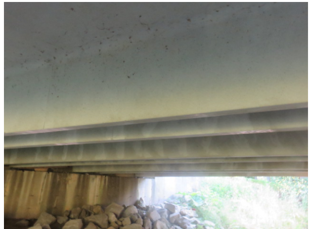
Underside of precast
