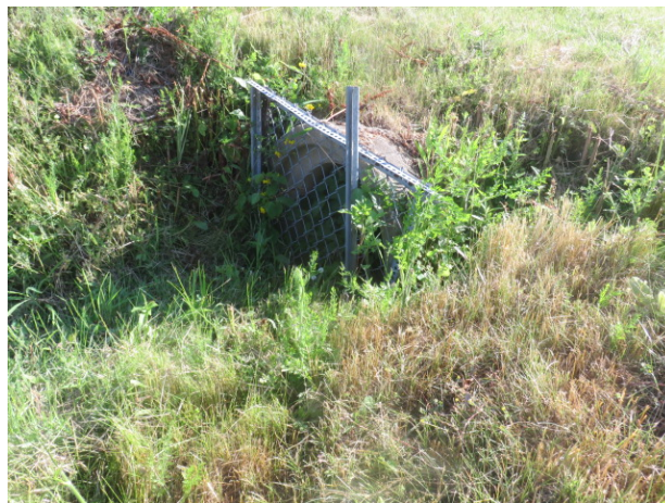
Pond outlet structure in good condition
