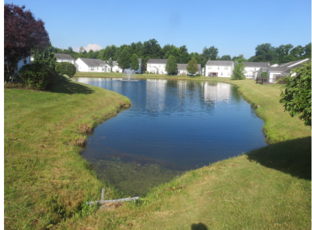
Pond, viewing west; note debris buildup in foreground
