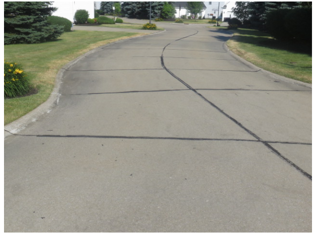
Concrete street and control joints in good condition
