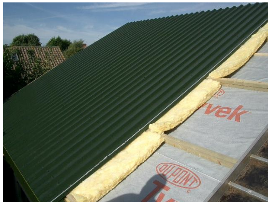
Scaffolding up and first sections of new roof being installed, showing fibreglass insulation
