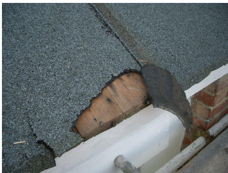
View of old roof, and close up of worn and torn leaking old roof felt
