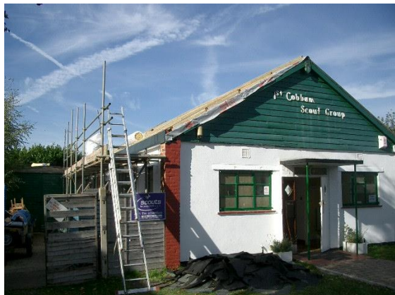
Scaffolding up and first sections of new roof being installed, showing fibreglass insulation
