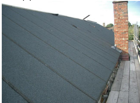
View of old roof, and close up of worn and torn leaking old roof felt
