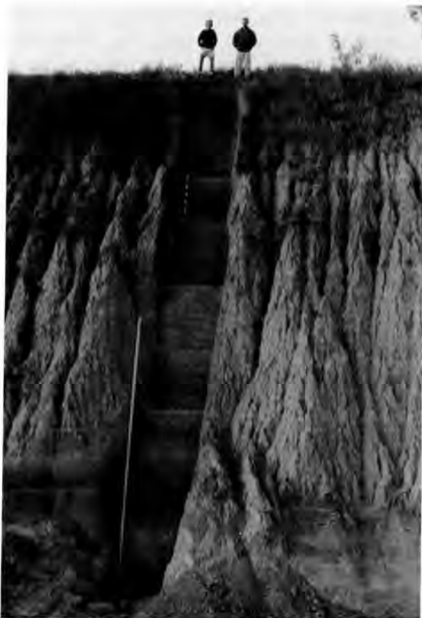
Figure 17. Photograph of the spillway trench wall.
