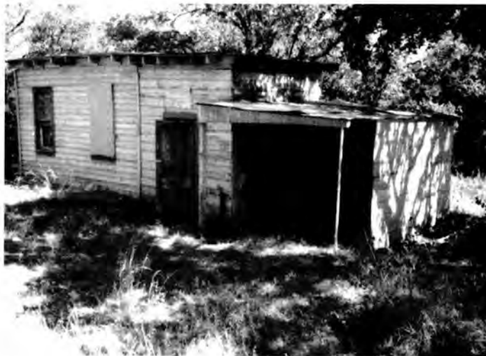
Figure 5. Building 13-A, cottage; west and south elevations.
