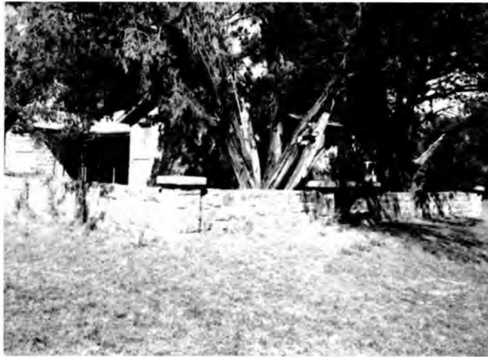
Figure 4. Building 13, cottage, front and east elevations;
