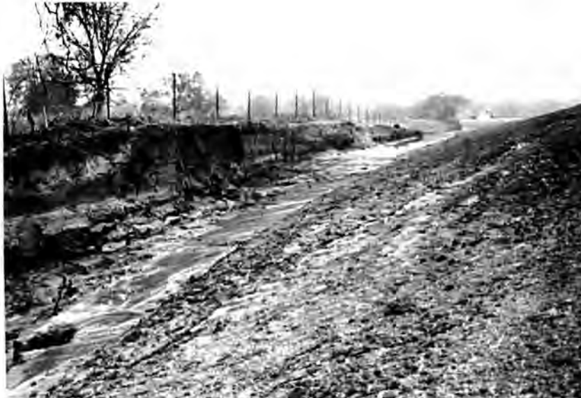
Figure 3. View from the right (south) bank of Smith Creek toward the south wall of the valley showing the long gentle taper of the levee from its crest (tree at left) toward the distant wall of the valley, the floor of the roadbed cut (left middle ground), the roadbed fill (right side of picture), and the vertical cut exposing the levee deposits (shovel indicates scale).
