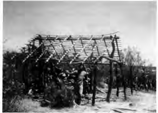
Figure 23. Abandoned jacal at 41SR48, dam area at Falcon Reservoir, 1950 photograph by Jack Hughes.
