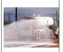
EnviroDust Suppress is a liquid water based protein colloid/polymer dust suppressant that combines wetting ability with a mixture of synergistic materials that enhance and extend the suppression of dust over time. Duration of dust suppression is dependent upon many factors including but not limited to the type of soil being treated, weather conditions, general climate and the amount of traffic on the area to be treated. EnviroDust Suppress is re-wetable and pliable.
