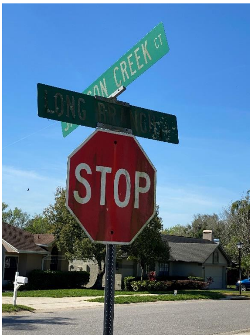
Figure 3 - Street Sign at the corner of Long Branch Ln and Jackson Creek Ct. - This top section of the sign is broken and is slumped at an angle and the bottom one is very dirty and the paint seems to be coming off.
