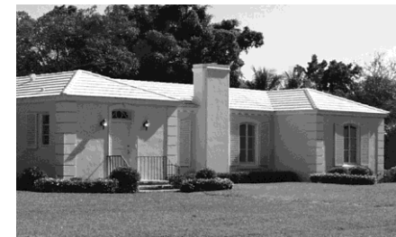
This chimney was stuccoed to match the surface treatment of the house.
