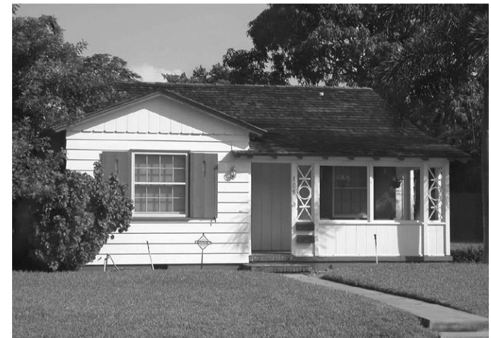
This residential structure is a contributing building in the Del-Ida Park Historic District in Delray Beach. The integrity of its original historic elements has been maintained.
