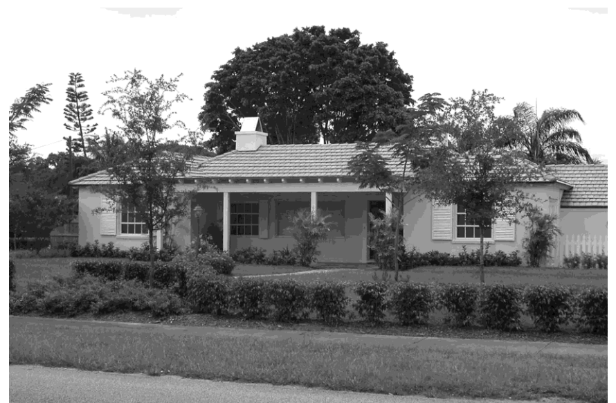
Masonry Vernacular residence
