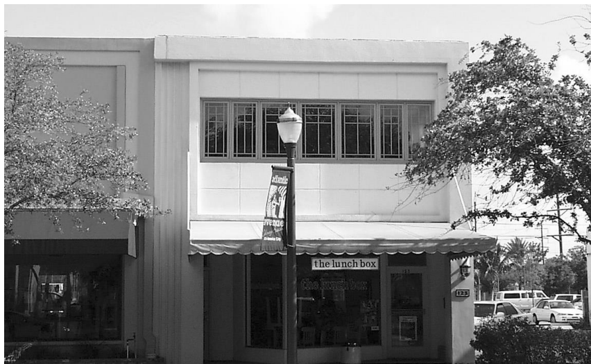
Masonry Vernacular commercial building
