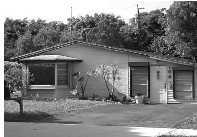
This residence is a non-contributing building to the Del-Ida Park Historic District because its age is not relevant to the period of significance, it has undergone severe window alterations and the carport has been enclosed.
