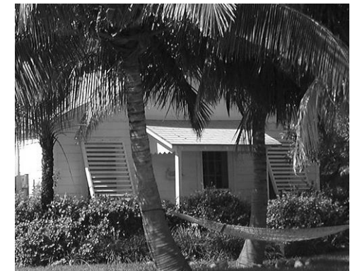
Visible impact to the character of the historic building should be considered when selecting a shuttering system.
