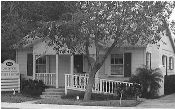
Example of a building retrofitted for access
