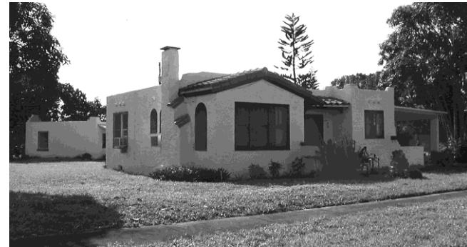
An accessory structure is visible behind this Mediterranean Revival residence.
