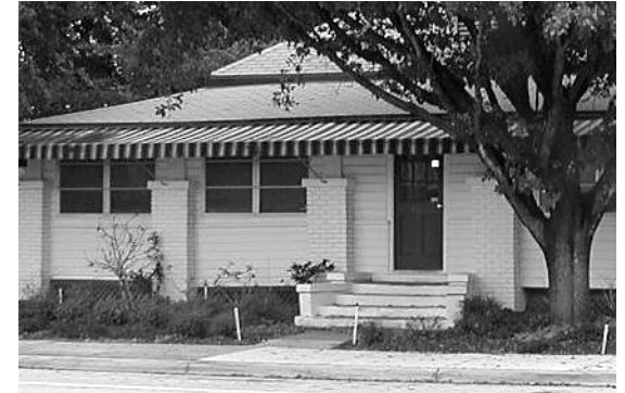
Example of a brick pier foundation
