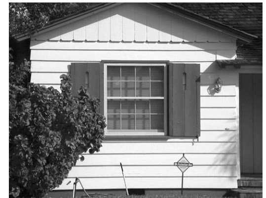
An example of properly installed shutters on a
