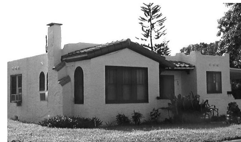
This Mission style house combines a gable roof of barrel tiles and flat roof. (Note that the chimney has elements of both the exterior surface and the roof.)
