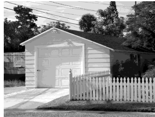
The most common example of an accessory structure is a detached garage that is associated with a residence, such as the structure at left.
