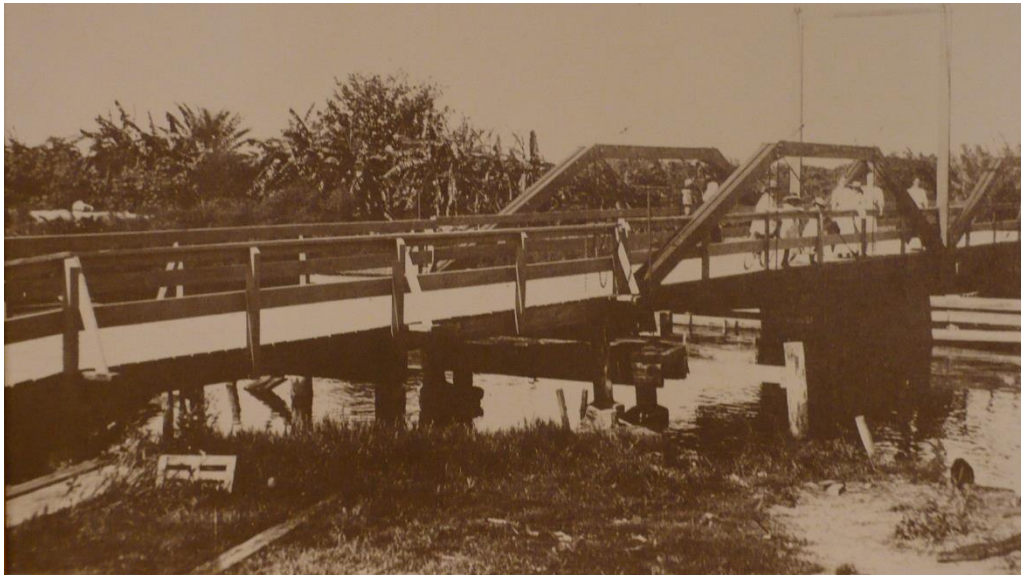
Atlantic Avenue Bridge, circa 1911. Photo courtesy City of Delray Beach.
