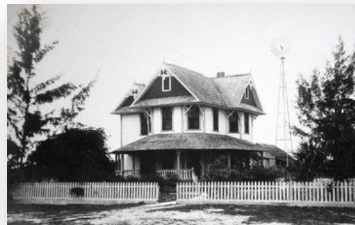
1902 Sundy House, built by Delray Beach's first mayor, John Shaw Sundy
