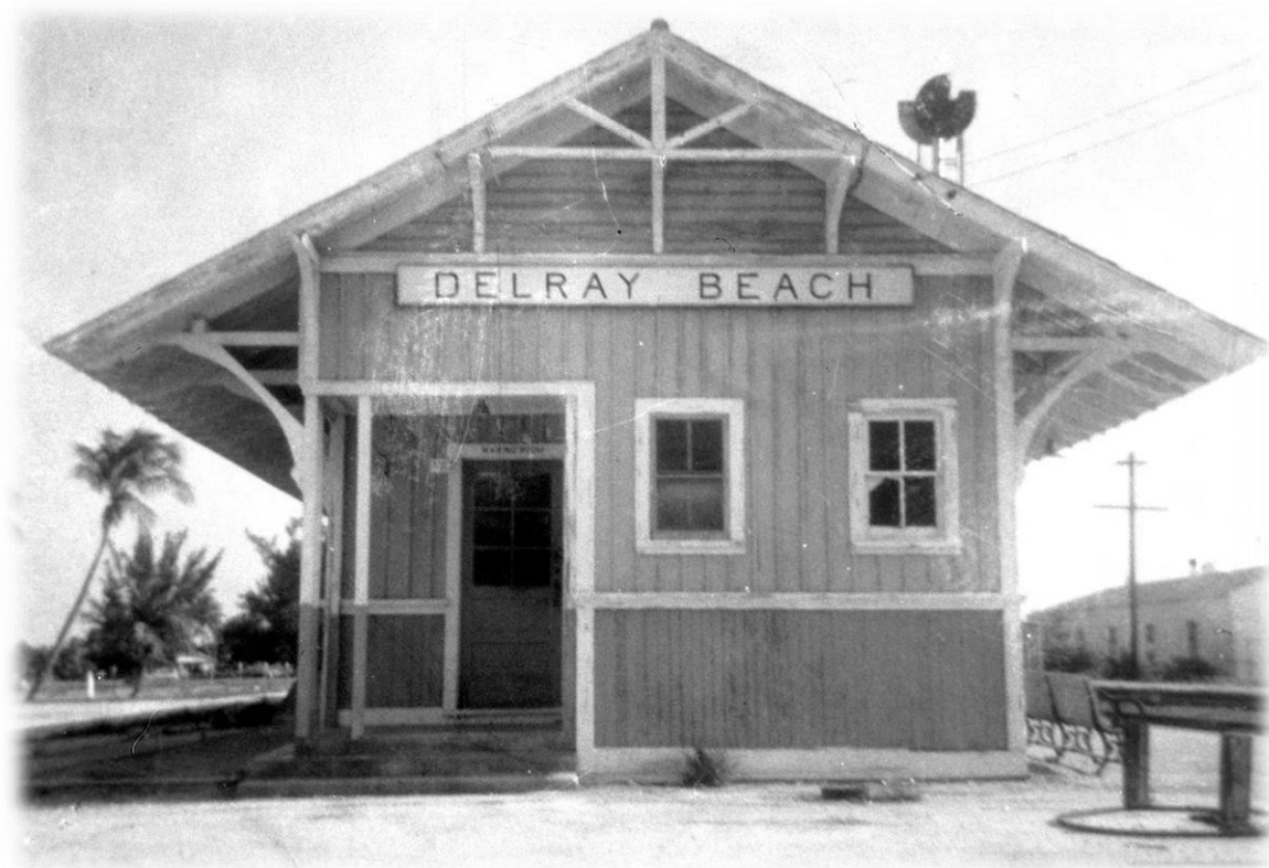
FIGURE 23. The Florida East Coast (FEC) Railway on Atlantic Avenue.
