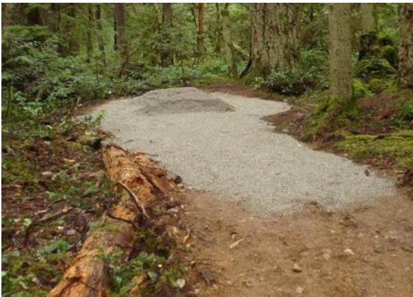
The first load at the end of the trail.
