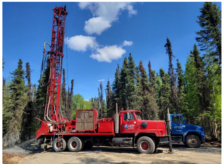
One of our road-access drill rigs with the pip truck behind it. We have two road-access drill rigs and two tracked rig drill rigs.
