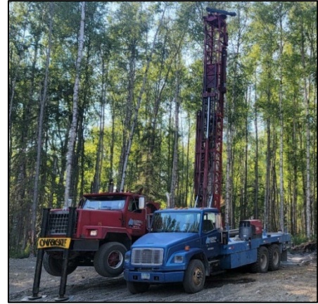
Our typical drill rig/pipe truck set-up.
