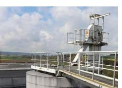
The Sitrans LR560 radarlevel transmitter can reliably and continuously determine the filling level of the cullet silo over the entire silo height.
