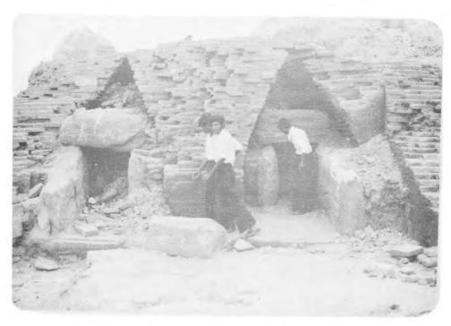
Twin Inlets With Gable Arch Containing a Granite Lined Water Duct
