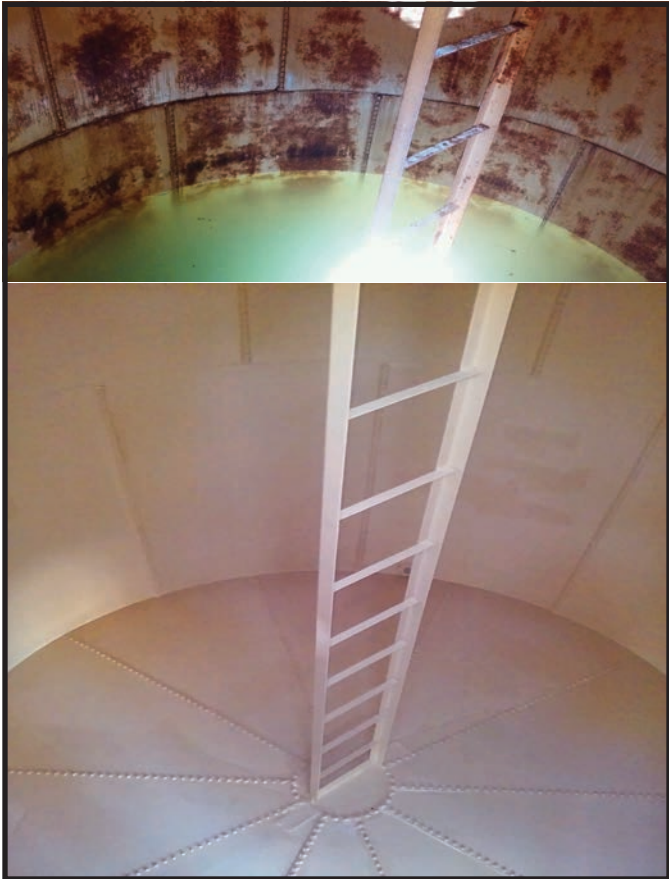
The old blue tank that TAHI acquired from the City of Zavalla was in bad shape with rust which prompted new sealing and painting inside. Thankful to our Operator Carl Pennington & Son for their work on our tank.
