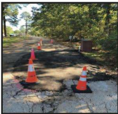
Road work at the gate entrance
