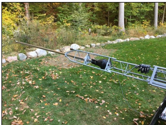
Original thrust bearing with rotator and mast installed.
