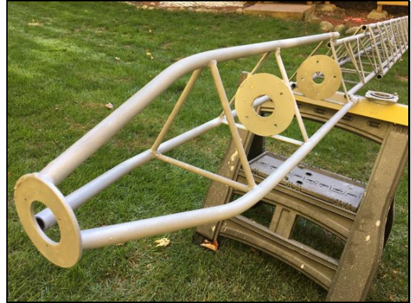
E-Z Way tower top section
