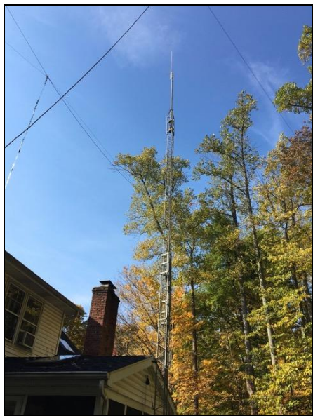
E-Z Way tower - cranked up for use with Diamond Dual-bander installed All Photo Credits: Tom Coury, WX1T
