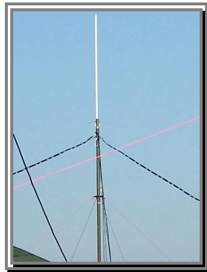
28 Ft. Mast with Dual-Bander and Skeleton Sleeve dipole Photo Credit: W1QK
