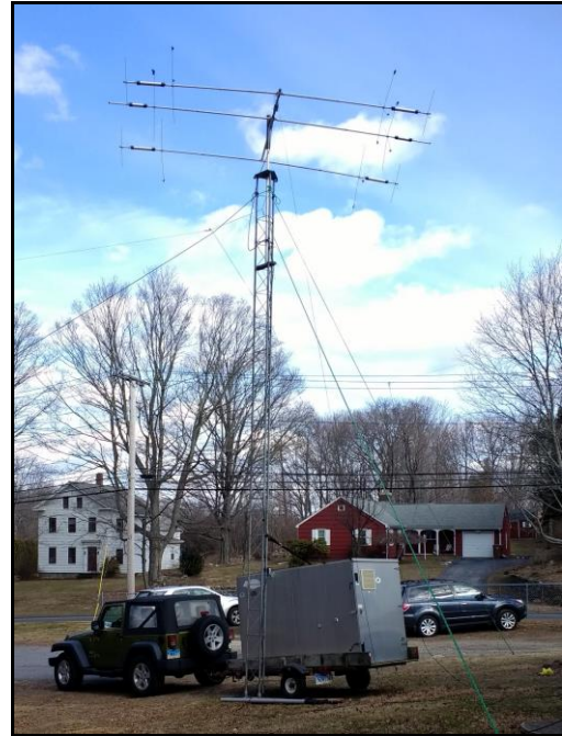
Portable tower and Tribander
