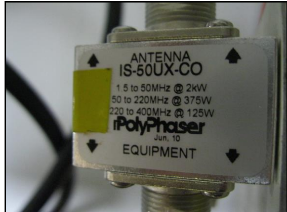
Polyphaser lightning suppressors are installed on each color-coded feedline.
