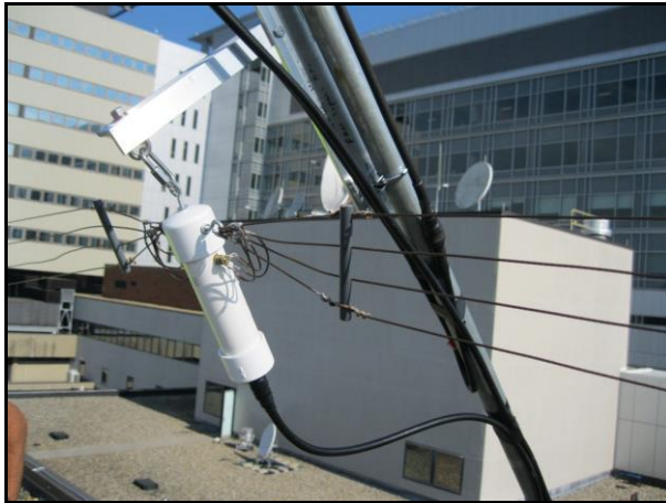
Fan dipole support bracket.
