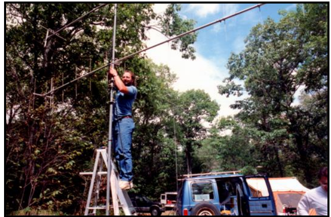
N1NRP installing the 144 MHz. Yagi on a 25 Ft. push-up mast.
