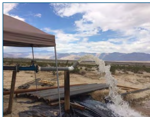
Well Development for the Rams Hill Water Supply Project
