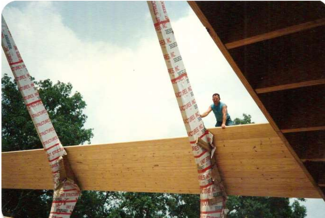
Working on the sanctuary roof
