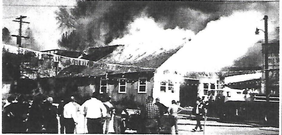
Rapid fire spread is evident.
