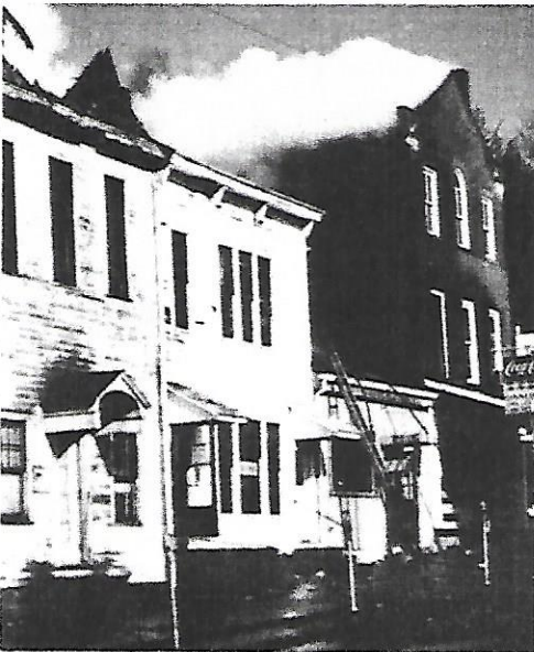
Fire spread through building
