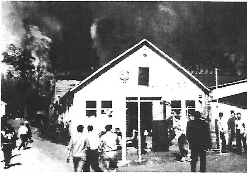
Moving equipment from building.
