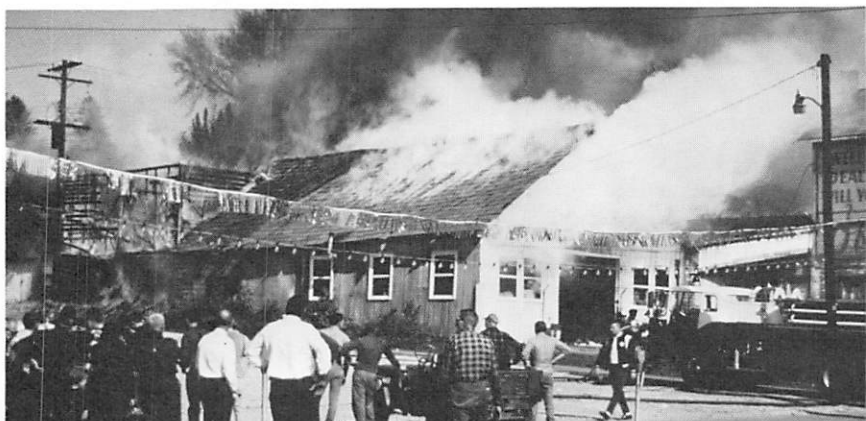
Rapid fire spread is evident.
