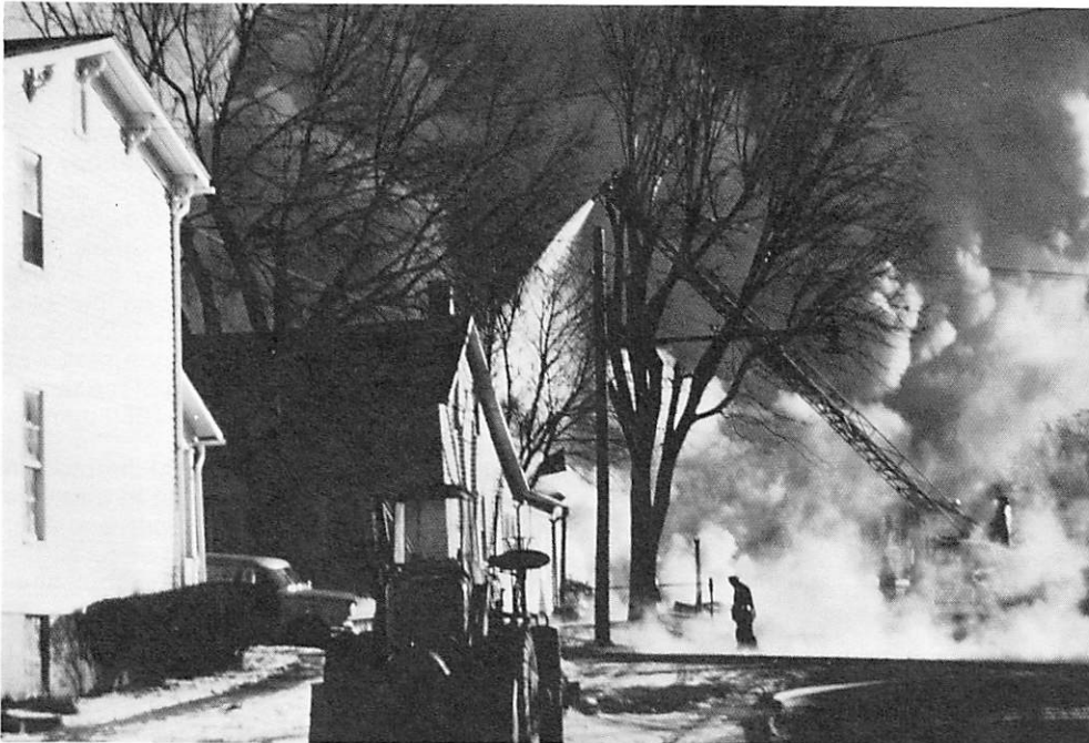
Jim & Bob's Implement fire. Aerial ladder played a major role in extinguishment.
