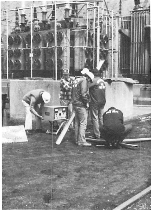
Morgan County Fire School Electrical Class — Ohio Power Plant 1979.
