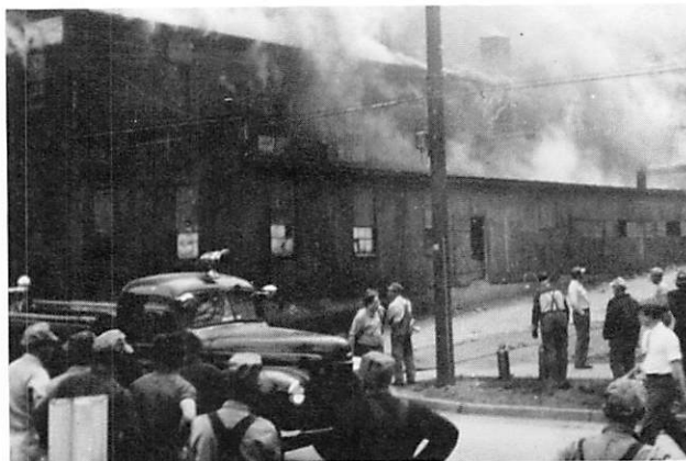
Brown-Manly Fire 1950. The blacksmith Shop was the origin of the fire.
