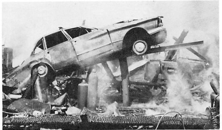
Service station fire at Gaysport in 1967.
