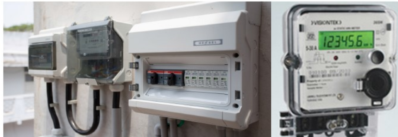
Net metering display screen showing units consumed by consumer
