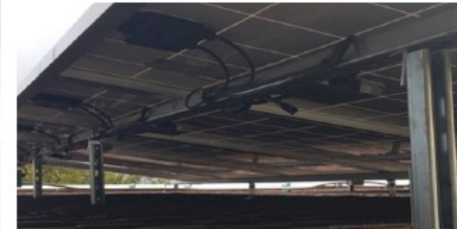
Correct cabling connection
