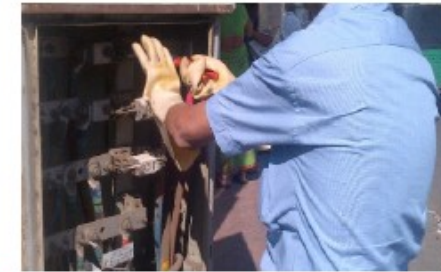
Correct practice - With safety gloves
