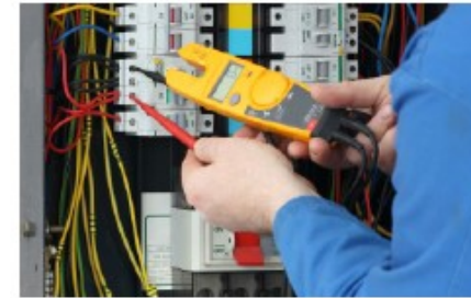
Incorrect practice - Without safety gloves
