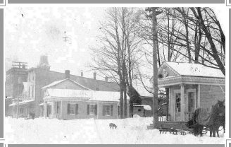
1905 Main Street Interlaken, Post Office & Banking House
