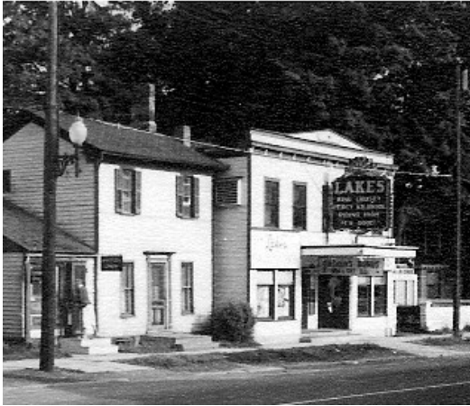
Original telephone office and the "Lakes" theater on Main Street.
