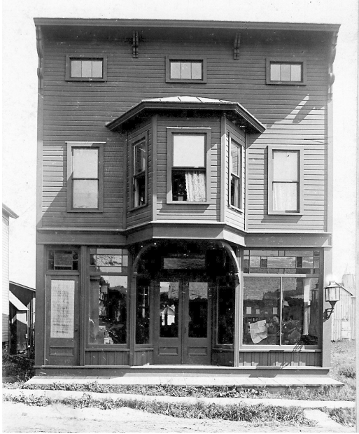
Review office on Railroad Avenue with its distinctive front façade ca 1893.
