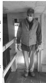
The short ceiling upstairs
