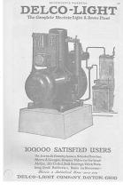
(DELCO) in 1909. By 1920, electric lights were common in cities, but not rural areas like Varick, New York. The first Delco-Light plant was a 750-watt, 32-volt unit (enough to light 37 20-watt bulbs). It was followed by a broad line of light plants with output up to 1,250 watts. In 1918 Delco-Light had a 3,000-watt light plant powered by a single-cylinder, 5 HP engine. By 1925 more than 60,000 Delco-Light plants had been sold.
