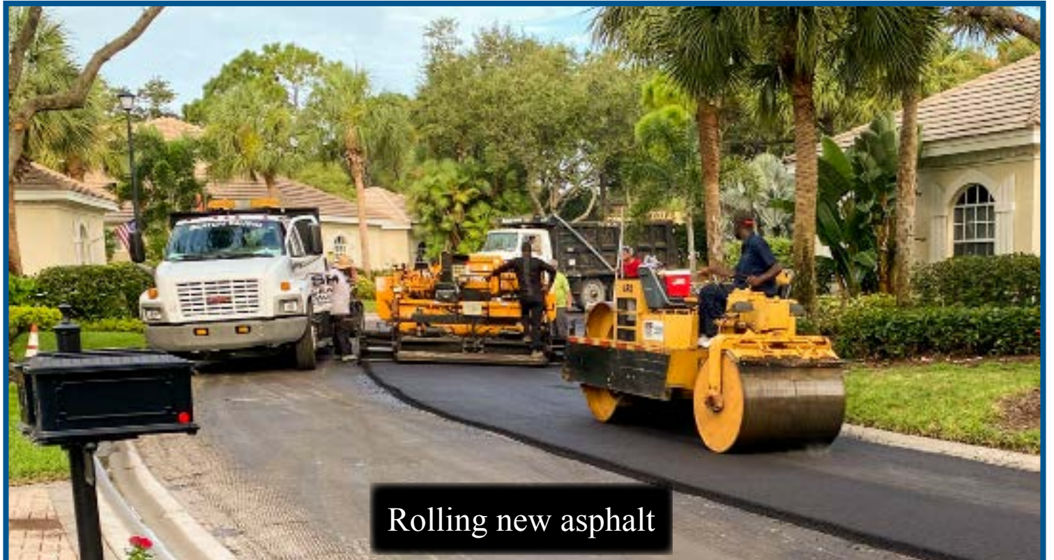
Laying new asphalt
