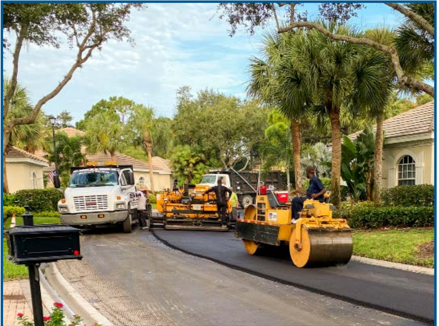
Olde Cottage Lane resurfaced
