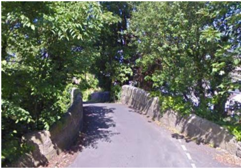
Photo 34. Canal Bridge on Hatlex
