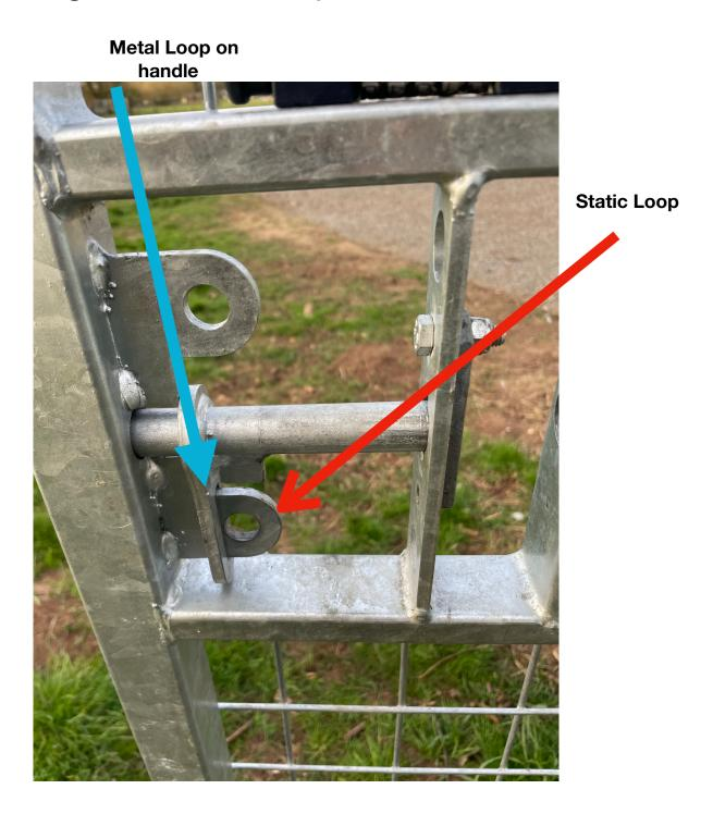
Place silver bar of padlock through static loop. \*\*Ensure the black knob of the padlock is facing you\*\*
